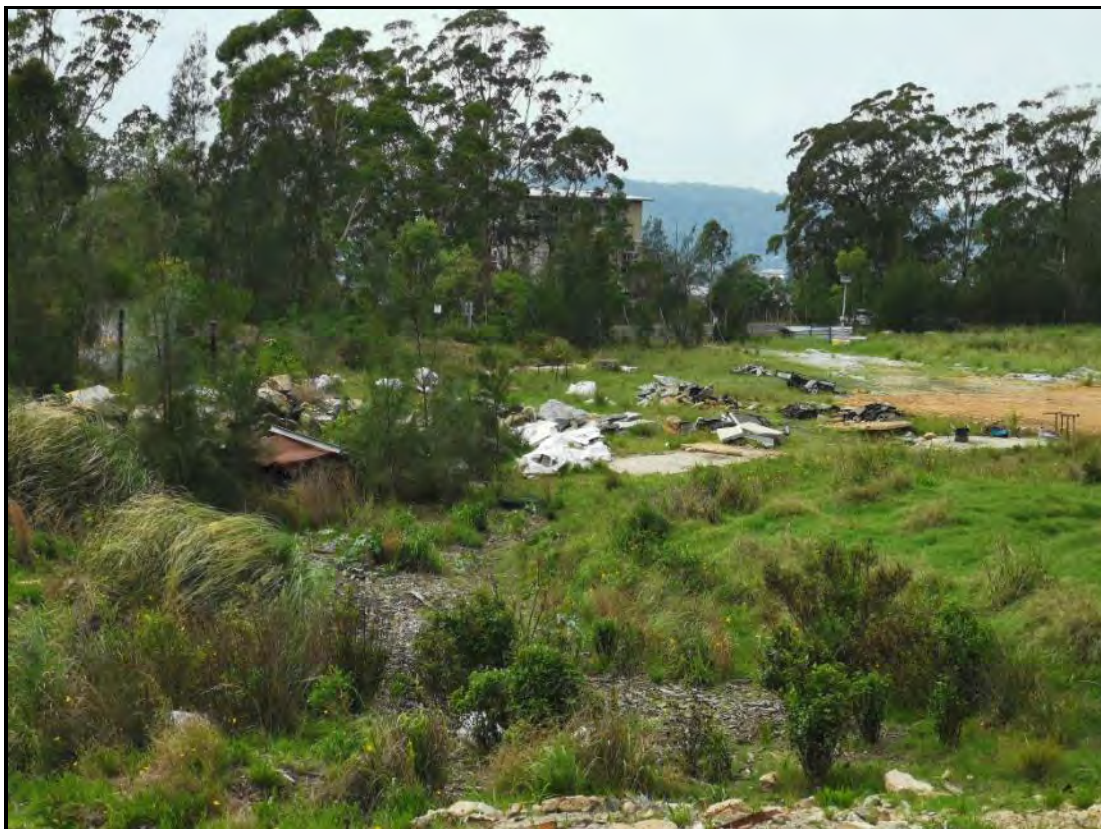
Photo 3. Cleared site area showing stockpiled building materials and dense exotic vegetation growth.
